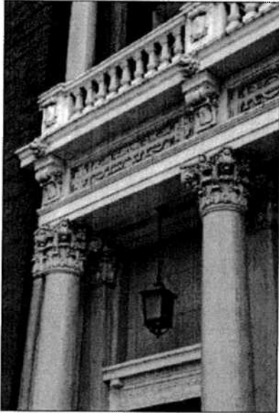
Ornamental details, such as those shown here above the entry, are delicately rendered in granite and terra-cotta. The ornament combines traditional Classical Revival elements with more modern, flat Sullivanesque and geometric decoration.
